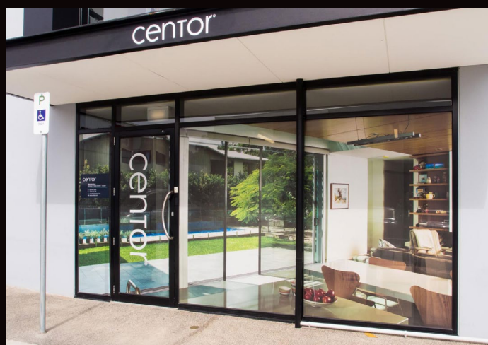
This is an example of a printed one way vision film. Note how the back layer is black to improve visibility from the inside.
